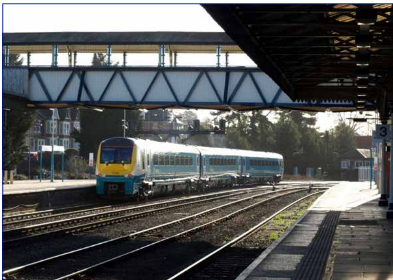
Hereford Barrs Court Station is a Grade 2 Listed building noted for its fine architectural features. The station buildings and footbridge are original, shown with an evening train departing for Cardiff.
